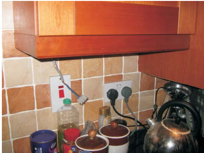
Electrical wiring in kitchen
