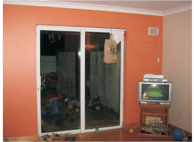
Hazardous pull cords to blinds
